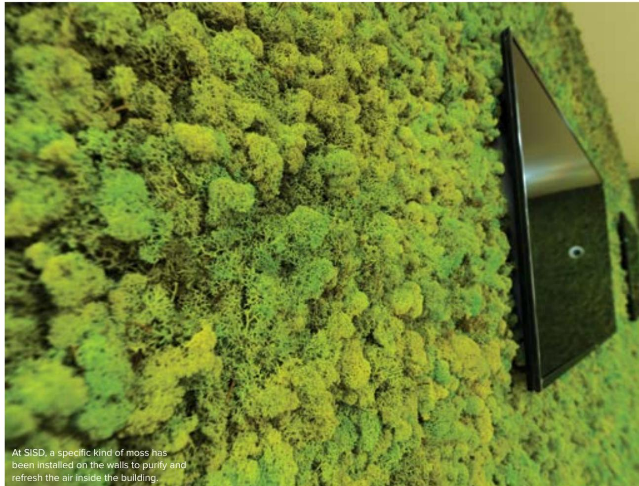
At SISD, a specific kind of moss has been installed on the walls to purify and refresh the air inside the building.
